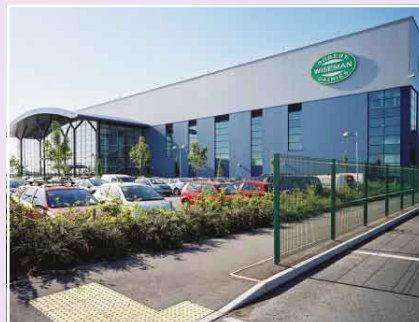
Robert Wiseman Dairies is using a reverse osmosis system from Elga Process Water to help meet its water use reduction target of 25% by 2015
