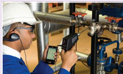
Marston’s Brewery has saved £60,000 (€70,000) in energy and hot water costs following installation of steam traps from Spirax Sarco
